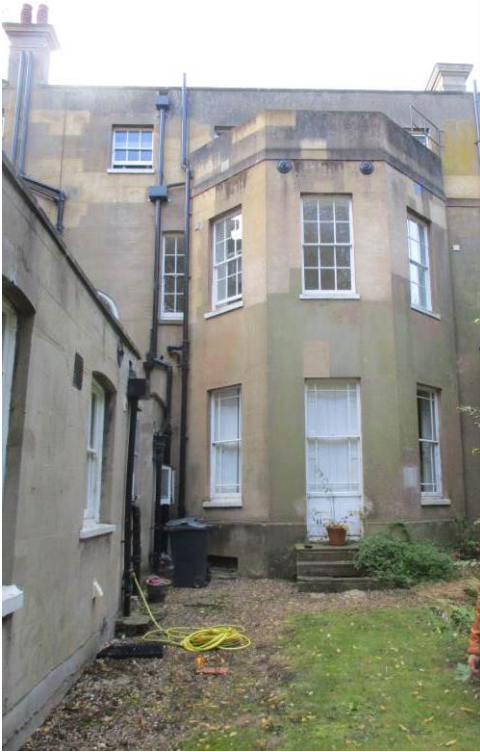
Site of light well to west elevation
