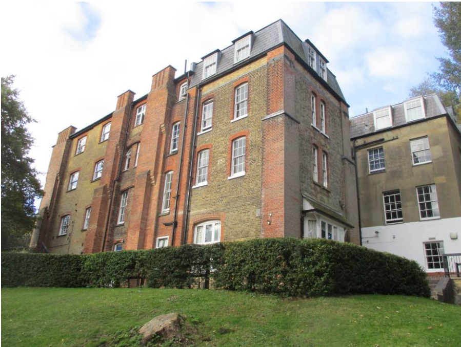
Later additions to building (east elevation)
